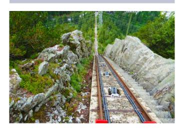
outer strands. This means that the required minimum breaking load of 850 kN has already been achieved through the outer strands alone and the intermediate strand layer offers additional breaking load, or in others words safety, for the operator. In internal testing, the entire rope achieved a breaking result of 45% above the required minimum breaking load. During the breakage testing, the conductivity of the electrical line was continuously monitored and none of the electrical lines showed any
